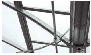
Rack & Pinion Gutter Vent
