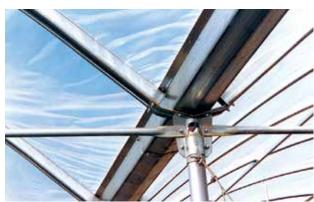
Super strength arch to gutter adapter
